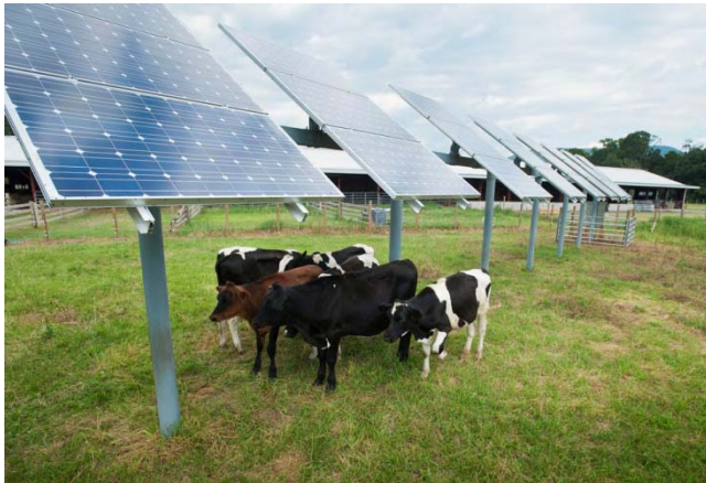
Umass Research Farm, South Deerfield 70 panel, 16.45 kW project installed in 2010
